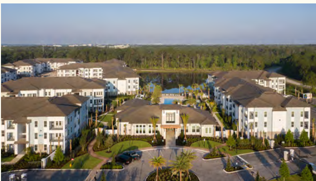
Drift at Town Center East Apartments
