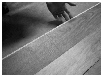
Fig. 6 – Locking long side with ends already locked.
