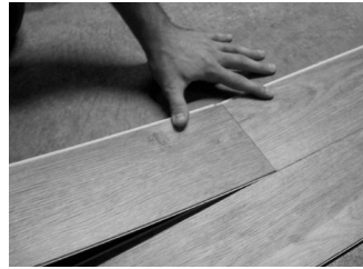
Fig. 5 – Angle end of next plank.
