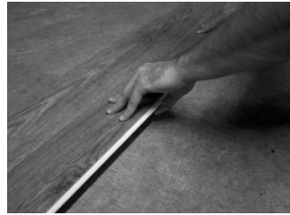
Fig. 4 – Angle long side into prior row.
